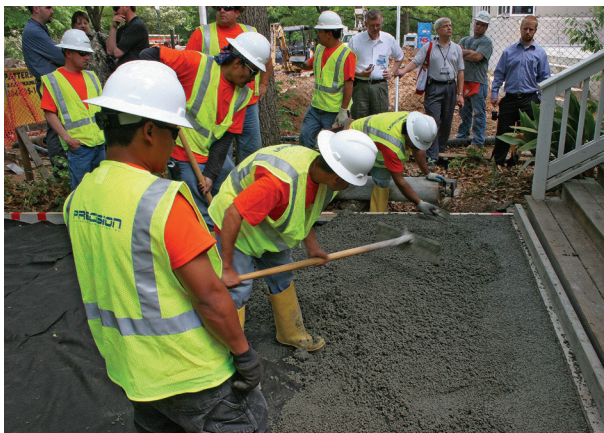
Placing pervious concrete with local labor.
