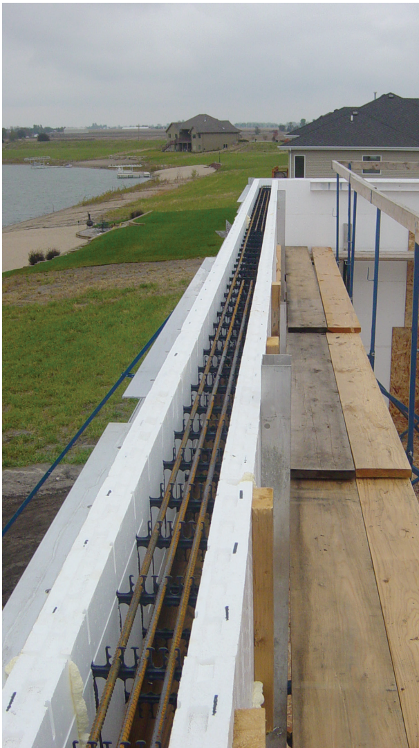
Insulating concrete forms being used in the construction of a walkout ranch home in Omaha, NE. Completed home, bottom photo (photos courtesy of Fox Blocks).
