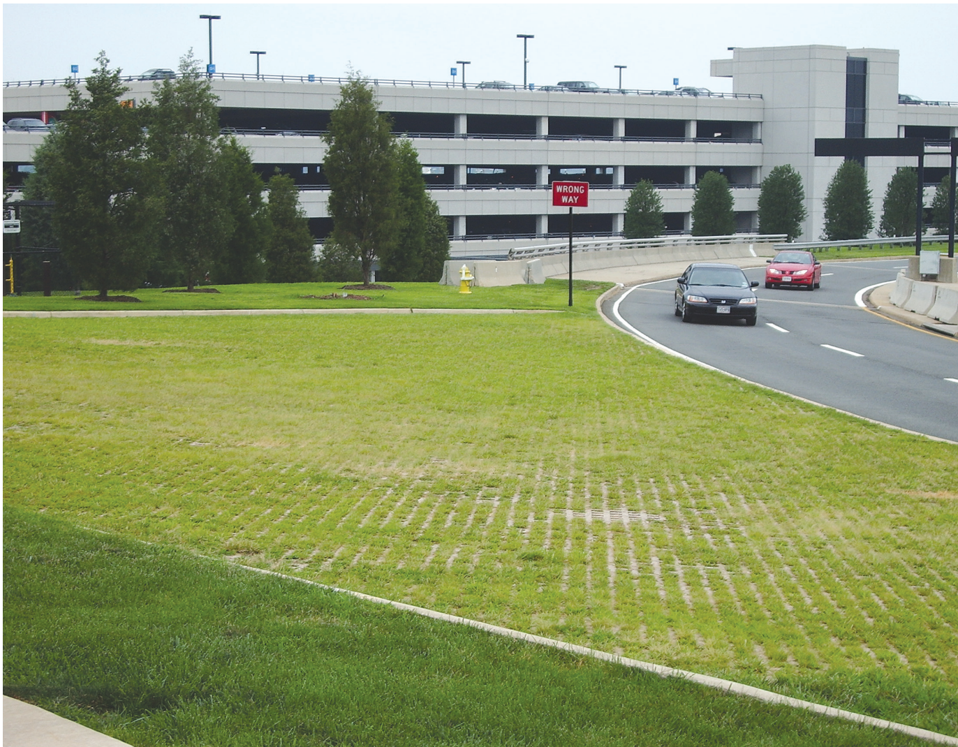
Fig. 2.28—(Top) Example of concrete grid pavement ( photo courtesy of Interlocking Concrete Pavement Institute ). (Bottom) Concrete grid pavements cover pull-over area near main terminal and concrete parking garage at Washington Dulles International Airport in Virginia ( photo courtesy of Interlocking Concrete Pavement Institute ).
