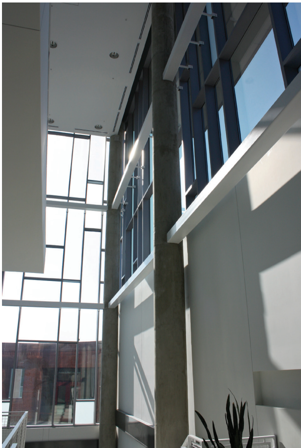
Fig. 2.13—Thermal mass with passive solar system. Building is located in Northern Minnesota and takes advantage of daylighting for solar gain and for occupant comfort while using thermal mass benefits from interior elements such as large exposed concrete columns.
