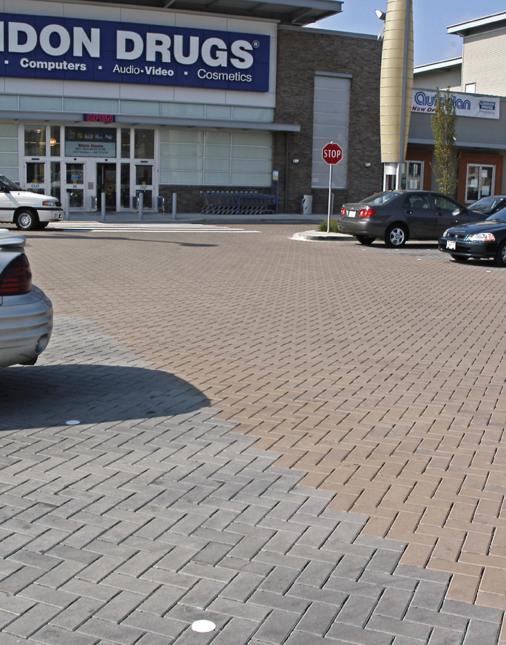
Fig. 2.29—(Left) Permeable interlocking concrete pavement manages roof and parking lot runoff at Marine Market Way in Burnaby, British Columbia (photo courtesy of Interlocking Concrete Pavement Institute). (Right) Residential development called Autumn Trails in Moline, IL, used permeable interlocking concrete pavement because it eliminated the need for a storm drainage system, thereby making permeable pavement cost-competitive with conventional asphalt (photo courtesy of Interlocking Concrete Pavement Institute).
