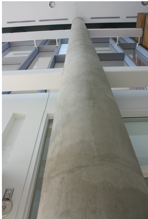
Fig. 2.13—Thermal mass with passive solar system. Building is located in Northern Minnesota and takes advantage of daylighting for solar gain and for occupant comfort while using thermal mass benefits from interior elements such as large exposed concrete columns.
