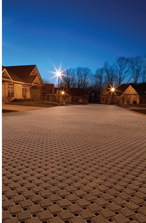
Fig. 2.29—(Left) Permeable interlocking concrete pavement manages roof and parking lot runoff at Marine Market Way in Burnaby, British Columbia (photo courtesy of Interlocking Concrete Pavement Institute). (Right) Residential development called Autumn Trails in Moline, IL, used permeable interlocking concrete pavement because it eliminated the need for a storm drainage system, thereby making permeable pavement cost-competitive with conventional asphalt (photo courtesy of Interlocking Concrete Pavement Institute).
