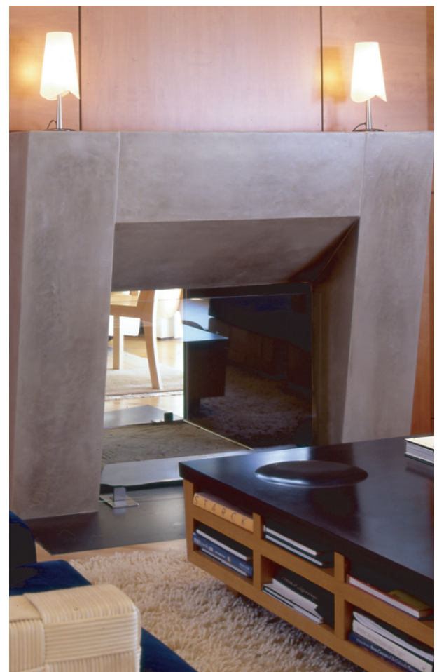
Fig. 2.5—Concrete fireplace through interior wall provides heat storage from thermal mass (photo courtesy of David Duncan Livingston/Buddy Rhodes Studio).
