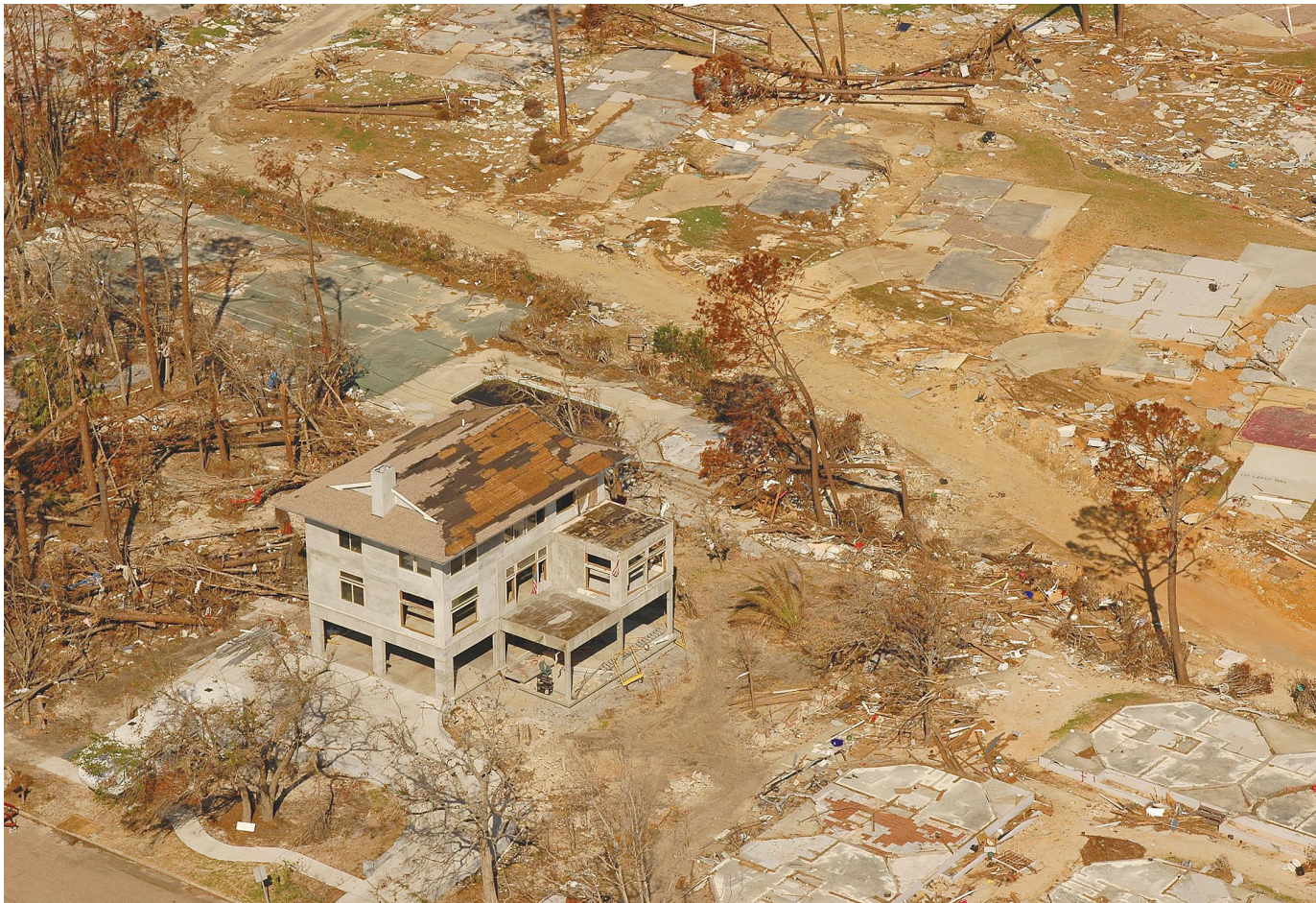
Fig. 2.39—Concrete home stands alone in Pass Christian, MS, after Hurricane Katrina in 2005. High water mark is 28 ft (8.5 m) up the structure (photo courtesy of John Fleck, FEMA).
