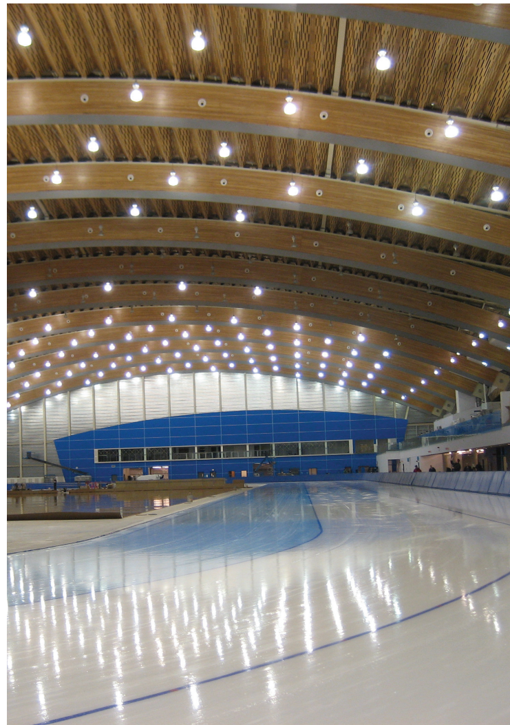
Richmond Olympic Skating Oval, built for 2010 Winter Olympics in Vancouver, BC, uses fly ash as cement replacement for parking slab, buttresses, shear wall, suspended slab, and activity slab (photo courtesy of Libe [John] Zhang).
