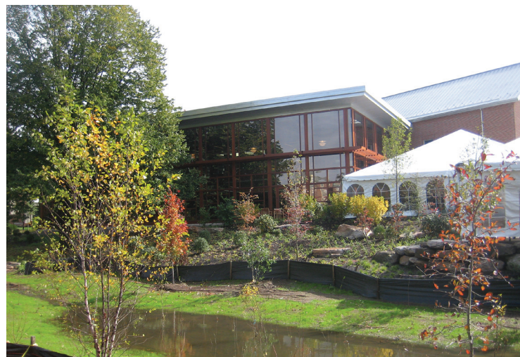
Fig. 2.22—Construction of six rain gardens at Mollie Dodd Anderson Library in Newtown, PA, makes collection of all site and building runoff possible, allowing water to infiltrate and recharge groundwater supplies as well as help to restore larger ecosystem of Neshaminy Valley (photo courtesy of Viridian Landscape Studio).
