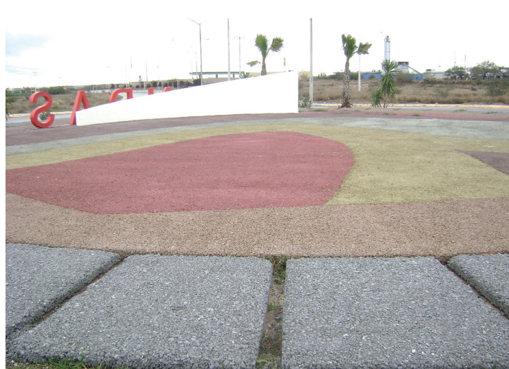
Fig. 2.23— (Top) Pervious concrete parking lot in Leawood, KS (photo courtesy of Concrete Promotional Group). (Bottom) Use of colored pervious concrete at entrance to Loma Real Housing Development in Reynosa, México, reduces maintenance and allows infiltration of rainwater (photo courtesy of Concrete and Cement Technology Center, CEMEX México).
