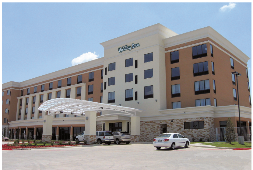
Autoclaved aerated concrete was used in the floor slabs, roof slab, and interior/exterior load-bearing walls during construction of this 126-room Holiday Inn hotel in Fort Worth, TX (photo courtesy of Xella Mexicana, S.A. de C.V.).
