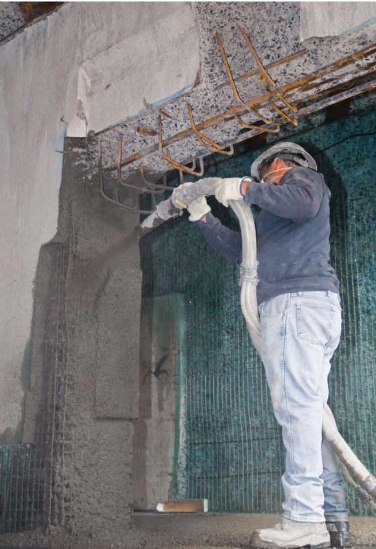
Fig. 4.7—Shotcrete being applied directly to the newly exposed surface without forming. Photo courtesy of American Shotcrete Association
