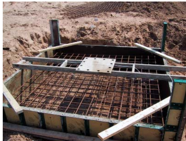
Fig. 1.24—Welded wire reinforcement placement in footing (Ice Mountain). Photo courtesy of ACI Committee 439 volunteers
