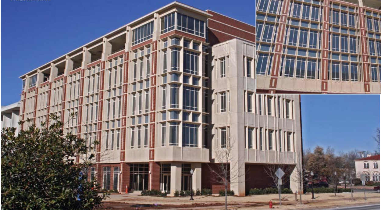
Fig. 3.10—Repetition of precast elements (Devon Energy Hall and Rawl Practice Facility, University of Oklahoma, Norman, OK). Photo courtesy of Architectural Precast Association
