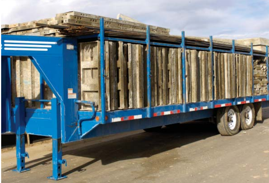
Fig. 2.15—In addition to the environmental benefits of reusing forms, substantial cost savings may be realized. Shown here are forms being reused between multiple job sites. Photo courtesy of Daniel Kourey
