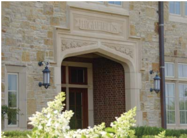
Fig. 3.17—This private residence incorporated a large amount of cast stone, which included a custom designed ornate door entry, window surrounds, water table, clad columns, roof coping, and site wall coping (Lewisburg Residence, PA). Photo courtesy of Cast Stone Institute
