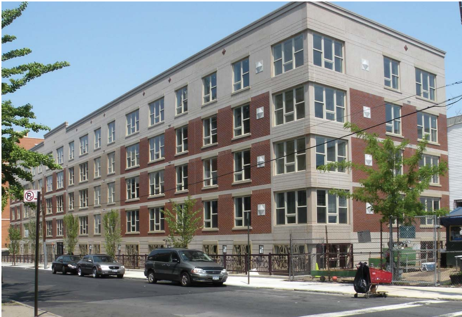
Fig. 3.71—Melrose Commons Site 5. Photo courtesy of Mike Smith, ALA Equus Designs
