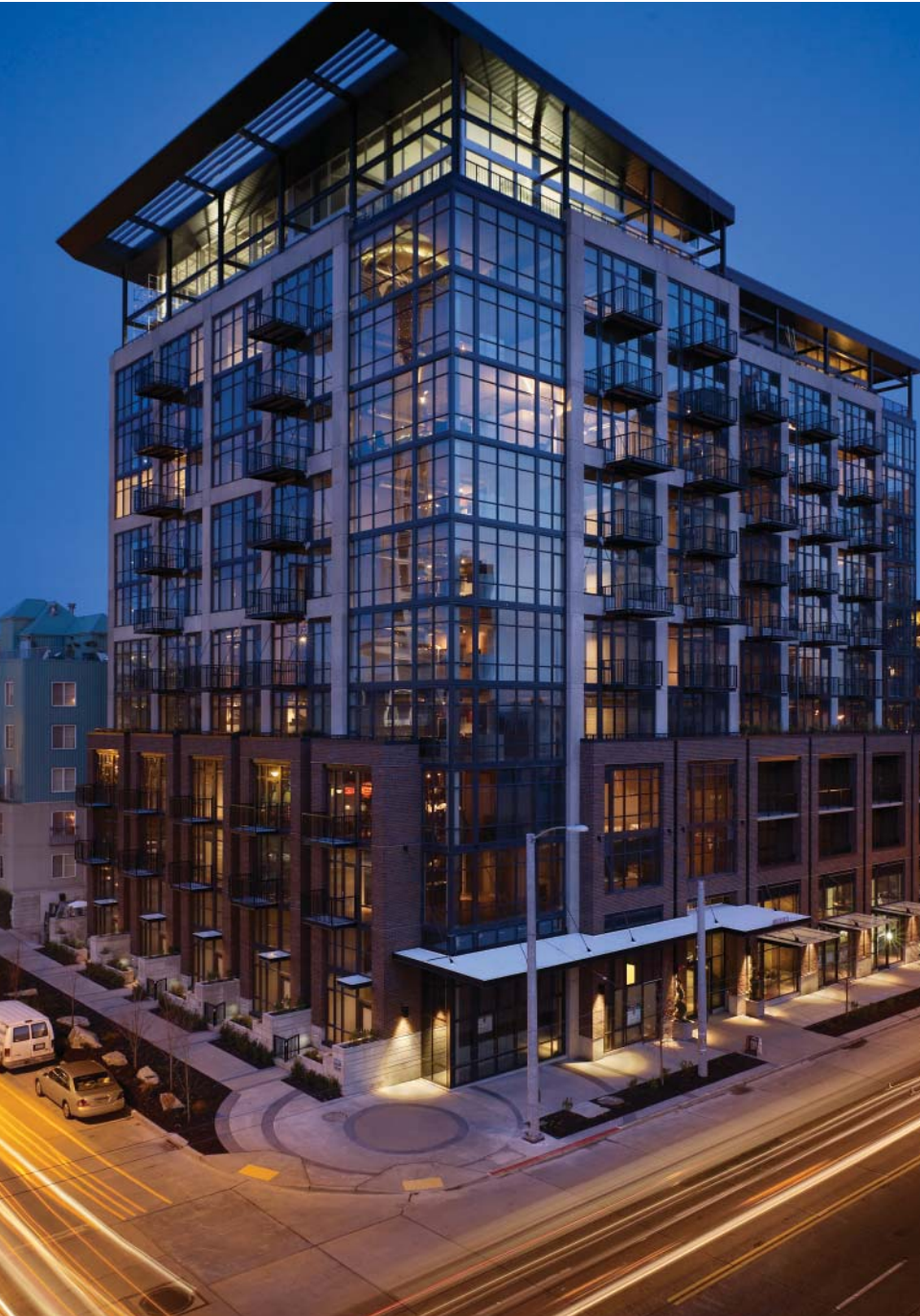
Fig 3.16—Cast-in-place concrete frame with post-tensioned flat-plate slabs are used in construction of the Mosler Lofts in Seattle, WA. Photo courtesy of Post-Tensioning Institute
