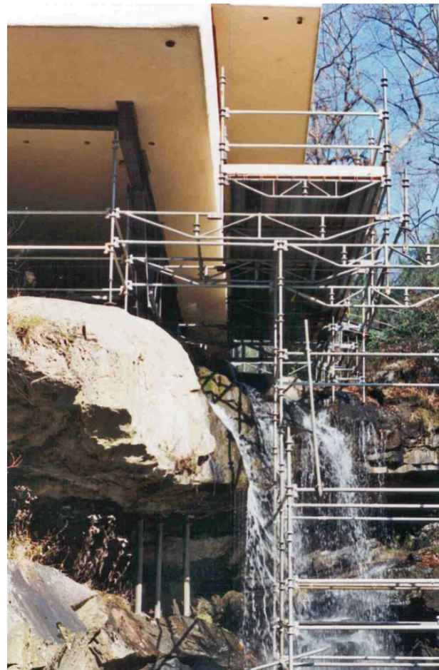
Fig. 4.16—Shoring of main terrace and additional shoring of cave below. Photo courtesy of Justin Brennan
