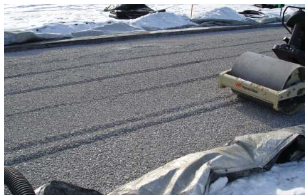
Fig. 3.31—Compaction equipment completes the base surface before placing the bedding layer. Photo courtesy of Interlocking Concrete Pavement Institute
