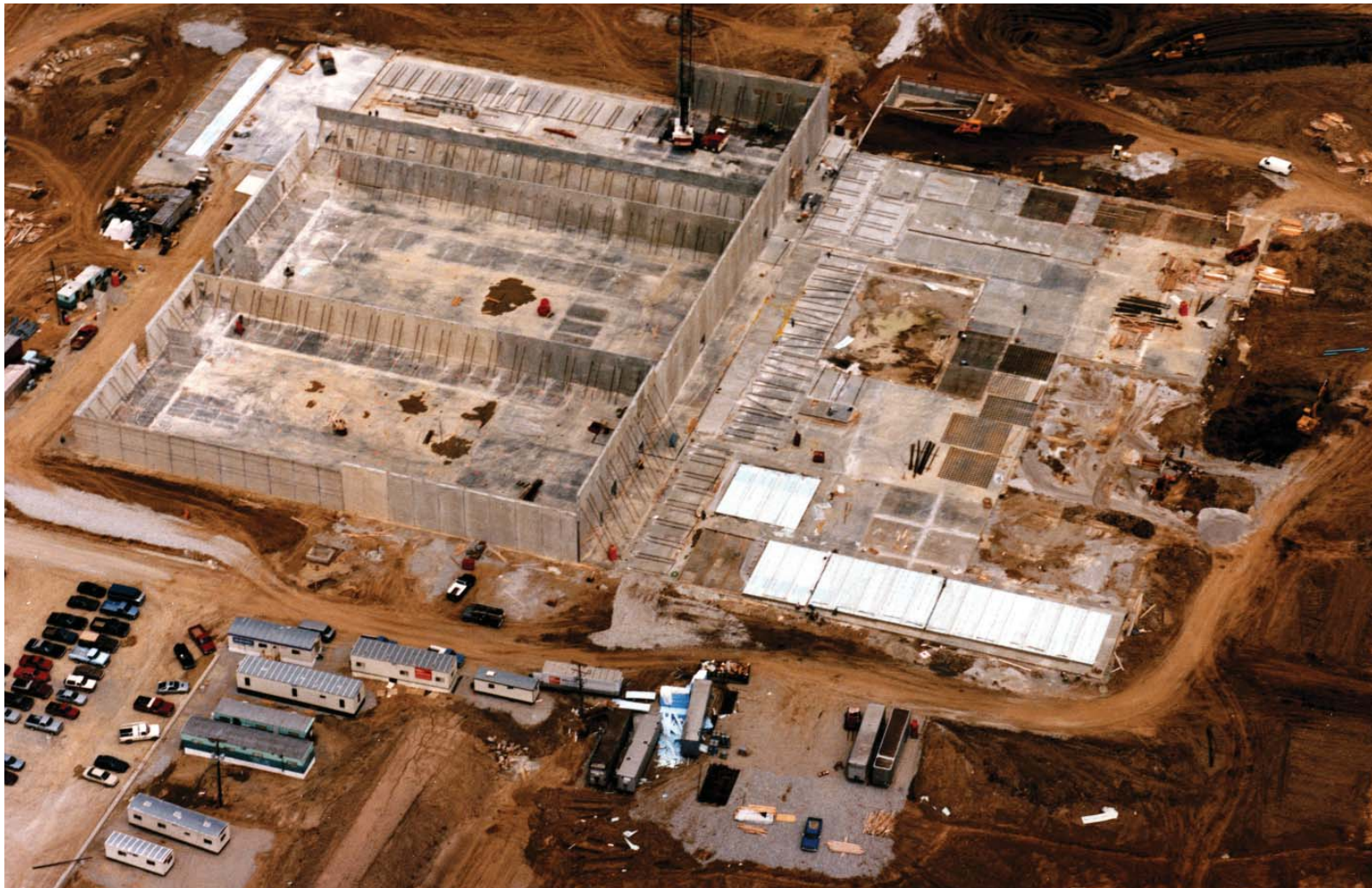
Fig. 3.81—Construction site with tilt-up panels during casting and erection. Photo courtesy of Tilt-Up Concrete Association
