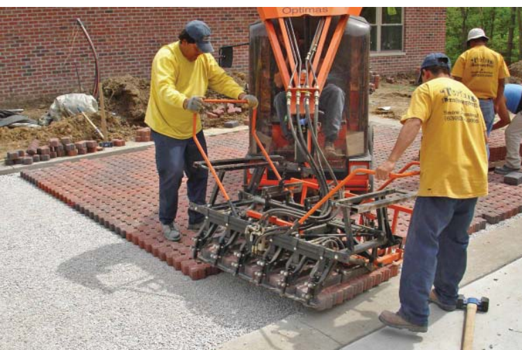
Fig. 3.34—Mechanical installation equipment places ready-made layers of the concrete pavers. Photo courtesy of Interlocking Concrete Pavement Institute
