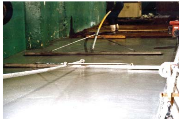
Fig. 1.14—Finishing the new transfer floor. Photo courtesy of Silica Fume Association
