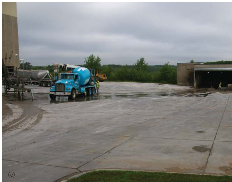
Fig. 1.2—Concrete trucks returning to deposit wash water: (a) trucks returning from a delivery have used self-contained washout. They are given wash water from the standpipe above the door and discharge into the weir system in the facility; (b) standpipe above doorway; and (c) not only is wash water treated, but also any water used to clean vehicles and rainwater is directed into the facility. Photos courtesy of Cemstone
