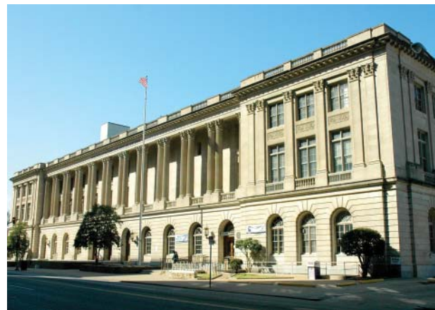
Fig. 4.18—University of Memphis' Cecil C. Humphreys School of Law following the renovation project. Photo courtesy of Lindsey Lissau
