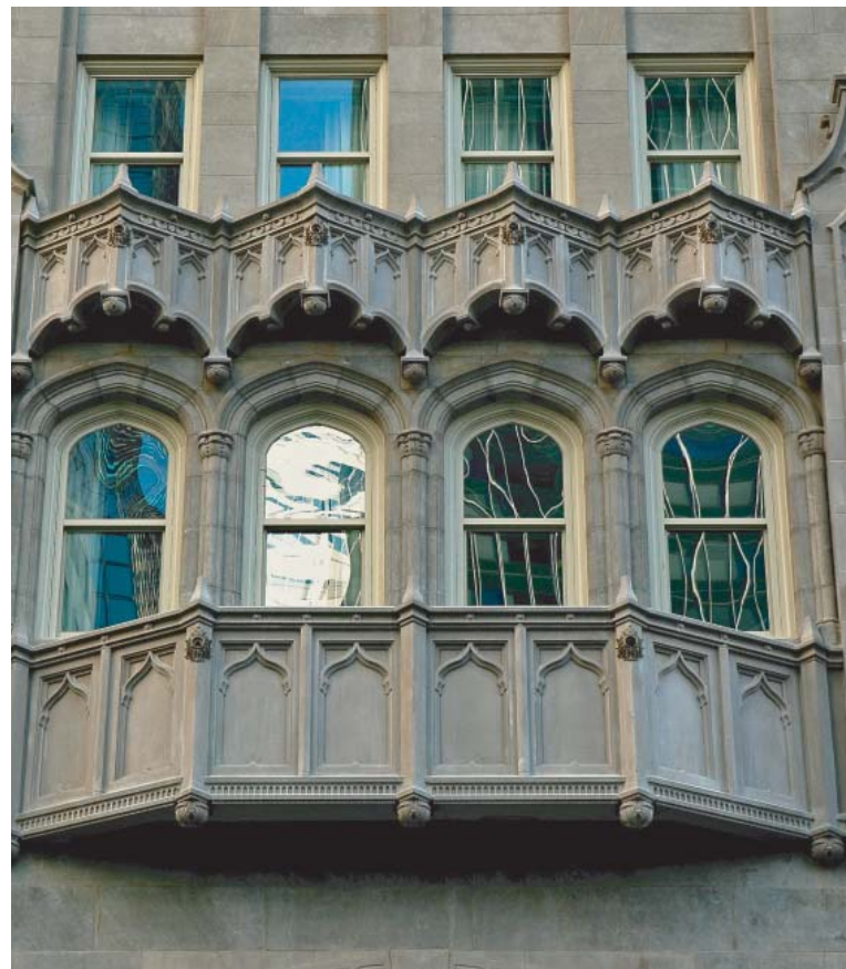
Fig. 3.20—Cast stone used in this collegiate-gothic style building with ornate window and door surrounds at The Taft School in Watertown, CT; and integration of new cast stone into the existing Joule Hotel, Dallas, TX, designed to appear as if it had always been an architectural element (Joule Hotel, Dallas, TX). Photo courtesy of Cast Stone Institute
