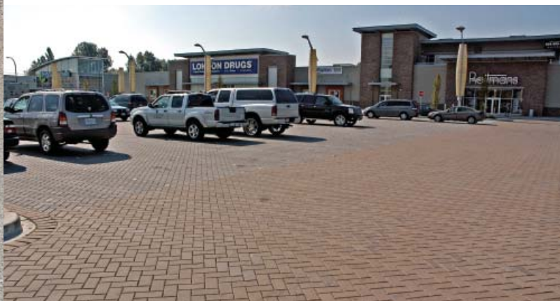
Fig. 3.37—Permeable interlocking concrete pavement manages roof and parking lot runoff at the Marine Market Way in Burnaby, BC, Canada. Photo courtesy of Interlocking Concrete Pavement Institute
