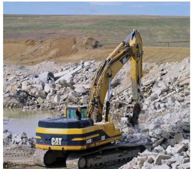
Fig. 1.20—Concrete from Denver’s former Stapleton International Airport was recycled and reused on site. Photo courtesy of Recycled Materials Company, Inc.
