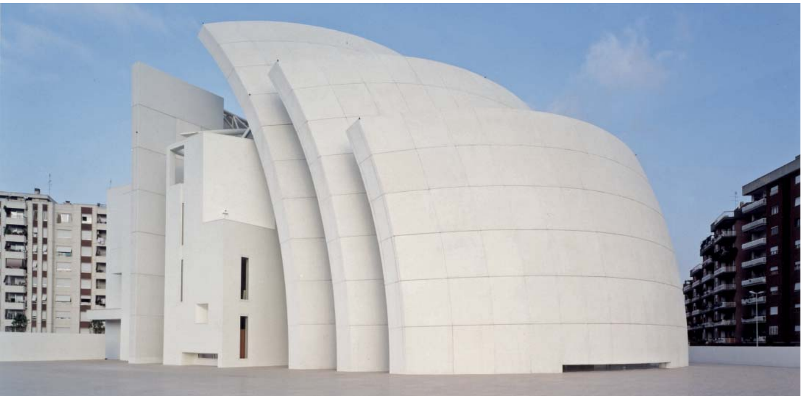
Fig. 1.29—Photocatalytic concrete was used at the Dives en Misericordia Church in Rome, Italy. Photo courtesy of Essroc Cement Corp.
