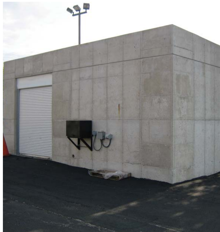
Fig. 2.13—Concrete X-ray vault consisting of 98% recycled materials. Photo courtesy of American Engineering Testing
