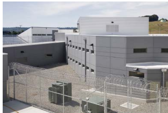
Fig. 3.73—Monroe Correctional Complex. Photo courtesy of Precast/Prestressed Concrete Institute
