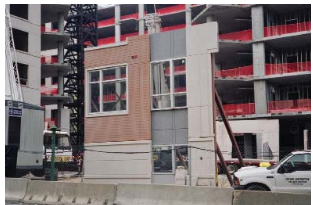
Fig. 3.15—A mock-up for the Domus project illustrates how color, texture, and special details can be combined in thin-shell precast concrete construction. Photo courtesy of National Precast Concrete Association
