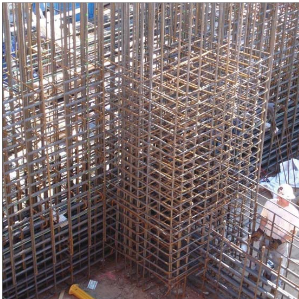
Fig. 1.23—Bar placement (Trump International Hotel & Tower). Photo courtesy of Skidmore, Owings, and Merrill LLP
