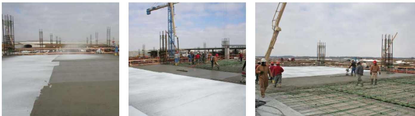
Fig. 1.16—Finishing operation. Photos courtesy of Silica Fume Association
