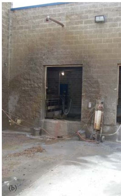
Fig. 1.2—Concrete trucks returning to deposit wash water: (a) trucks returning from a delivery have used self-contained washout. They are given wash water from the standpipe above the door and discharge into the weir system in the facility; (b) standpipe above doorway; and (c) not only is wash water treated, but also any water used to clean vehicles and rainwater is directed into the facility. Photos courtesy of Cemstone
