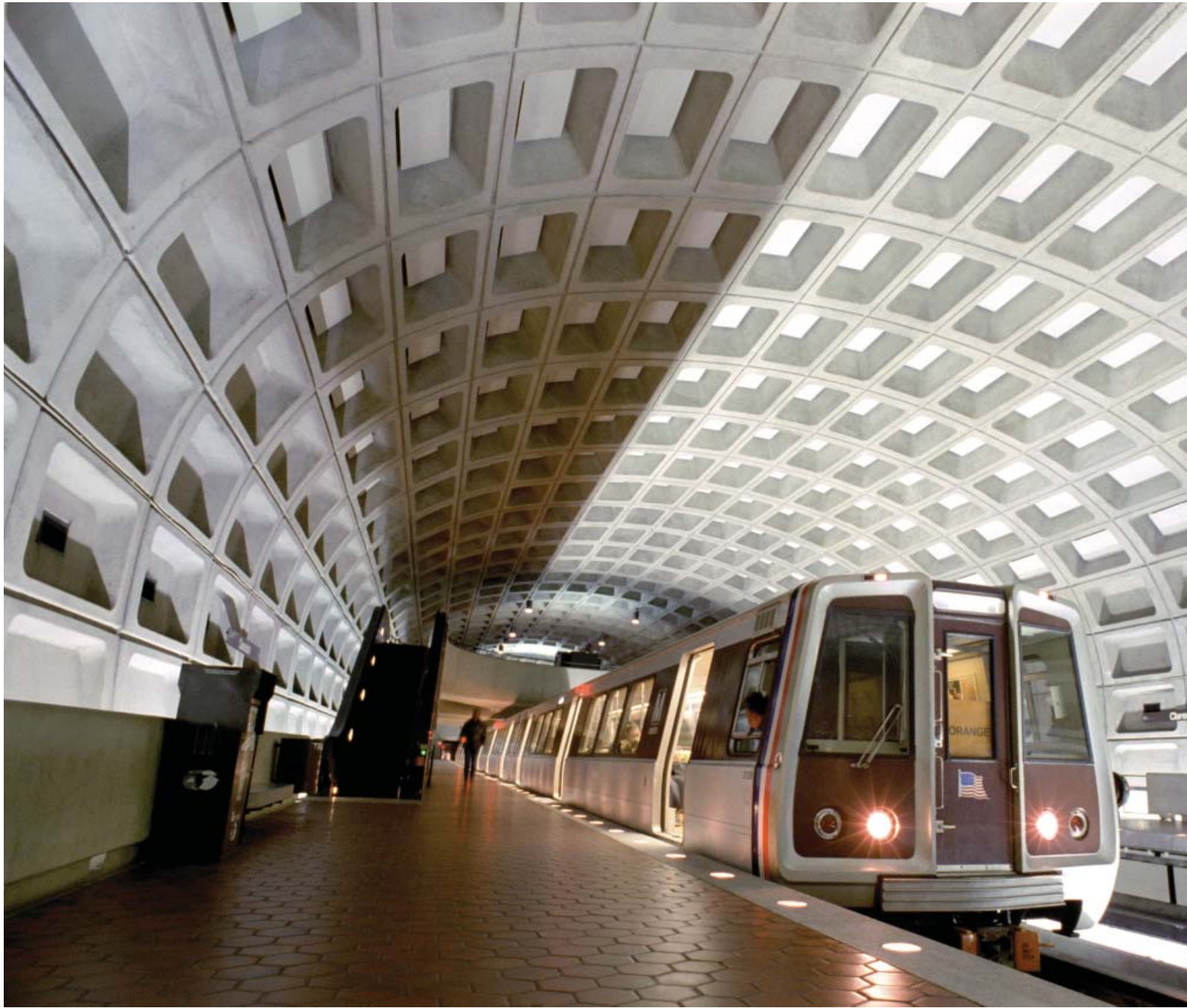
Fig. 2.14—Using waffle-formed concrete to form an architectural feature at the Washington, DC Metro. Photo courtesy of Kenneth C. Zirkel
