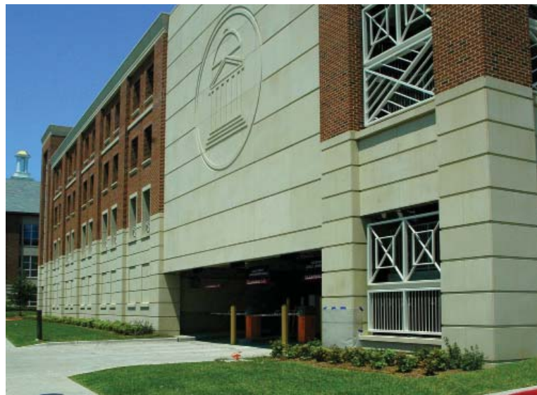
Fig. 3.5—Customized detailing (Southern Methodist University Parking Garage No. 7, Dallas, TX). Photos courtesy of Architectural Precast Association
