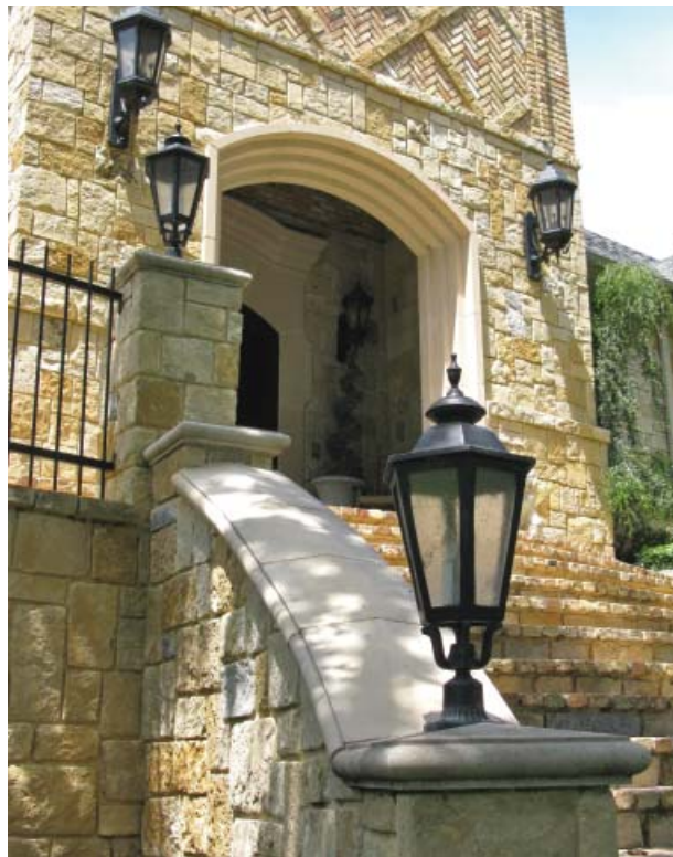
Fig. 3.19—Cast stone is used on the main entry porch of this grand residence and as wall capping (Green Residence, Mansfield, TX). Photo courtesy of Cast Stone Institute
