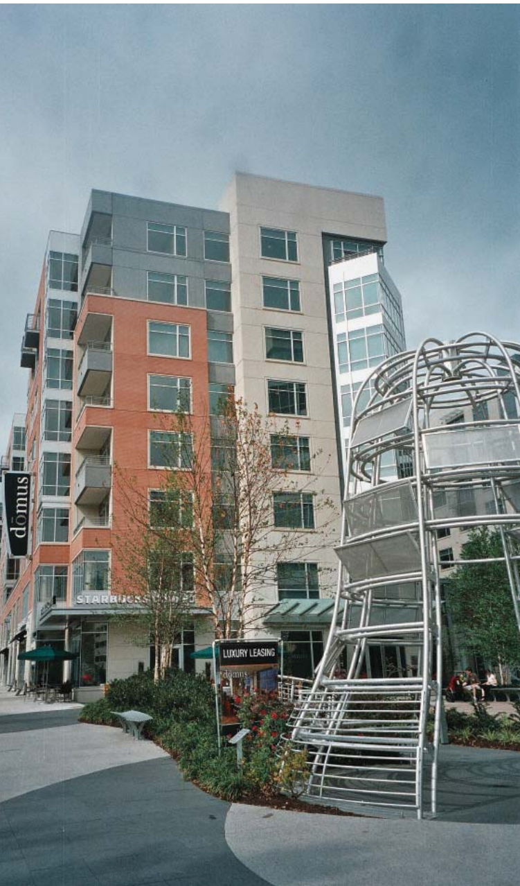
Fig. 3.13—Domus residential complex in Philadelphia, PA. Photo courtesy of National Precast Concrete Association
