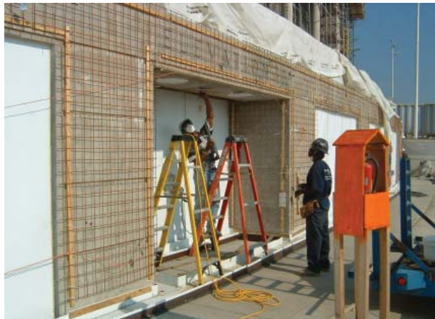
Fig. 4.10—Installation of realkalization system. Photo courtesy of International Concrete Repair Institute
