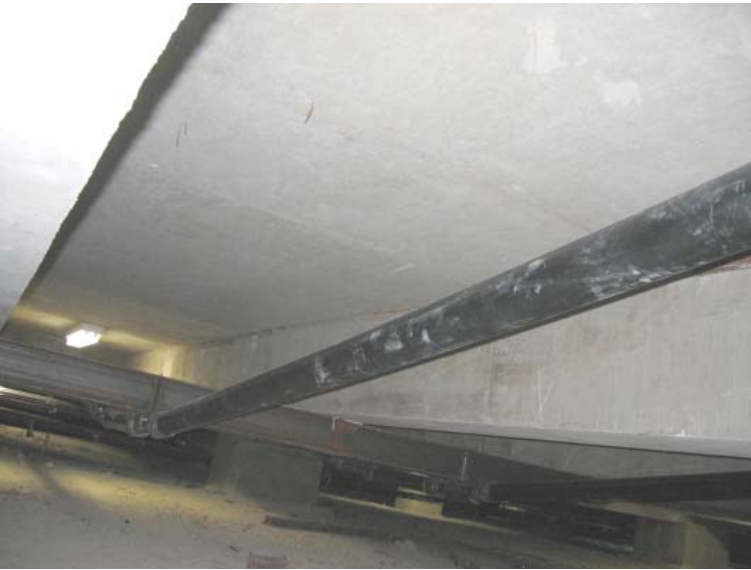
Fig. 4.6—External post-tensioning for strengthening concrete beams. Photo courtesy of VStructural, LLC (VSL)
