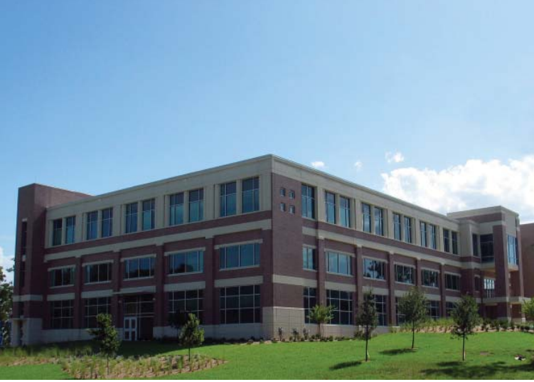
Fig. 3.12—University of North Florida Social Sciences Building. Photo courtesy of Architectural Precast Association
