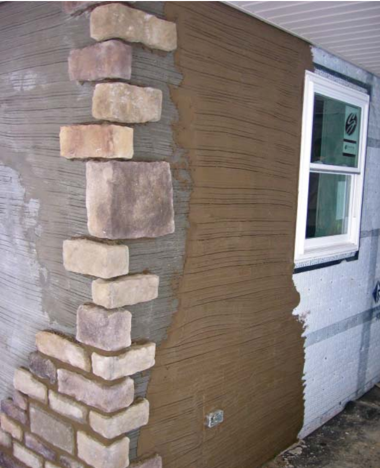
Fig. 3.47—Stone being laid directly over ICF. Photo courtesy of Insulating Concrete Form Association
