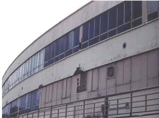
Fig. 4.9—Deteriorated concrete condition before completion of the work (Terminal A at Ronald Reagan Washington National Airport). Photo courtesy of International Concrete Repair Institute
