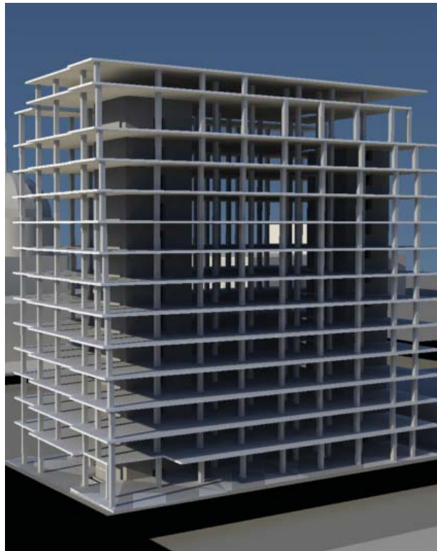
Fig. 2.12—Core walls within full structural system. Rendering courtesy of Webcor Builders
