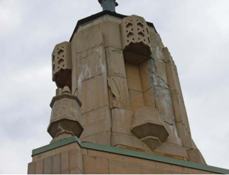
Fig. 3.21—Restoration (before and after): cast stone was used to replicate the entire original exposed aggregate structure, while maintaining the historical integrity of the intricate architectural details (Naples Central School District Naples, NY). Photo courtesy of Cast Stone Institute
