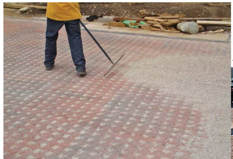
Fig. 3.36—The paver openings are filled with the small stones (CA-16), and excess stones are removed from the paver surface before compaction. Photo courtesy of Interlocking Concrete Pavement Institute
