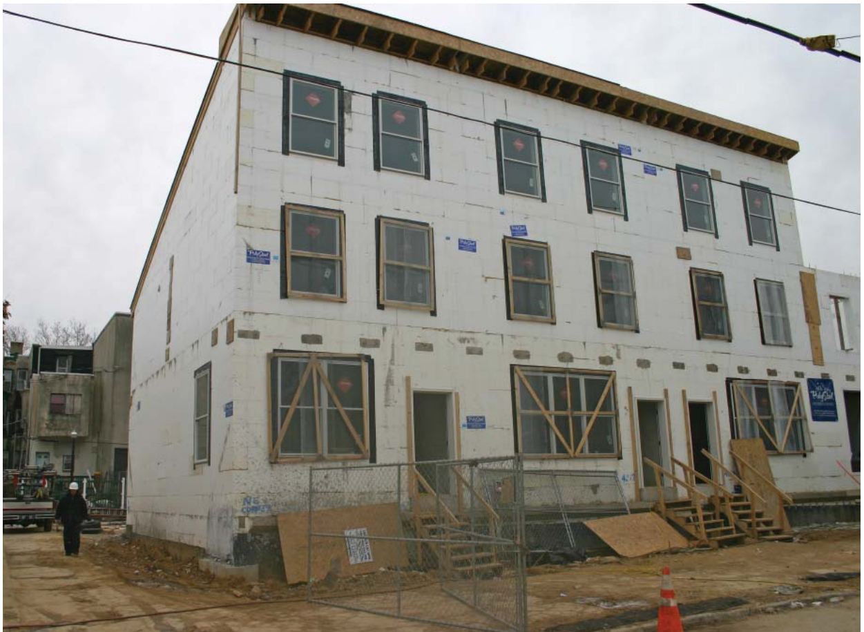
Fig. 3.50—Insulating concrete forms (ICFs) were selected for this project for their energy efficiency, durability, and safety. Photo courtesy of Portland Cement Association
