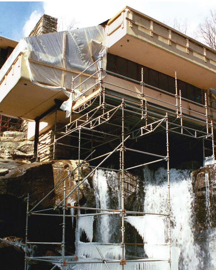
Fig. 4.15—Frank Lloyd Wright’s Fallingwater before retrofit. Photo courtesy of James Loper and Jason Hughes
