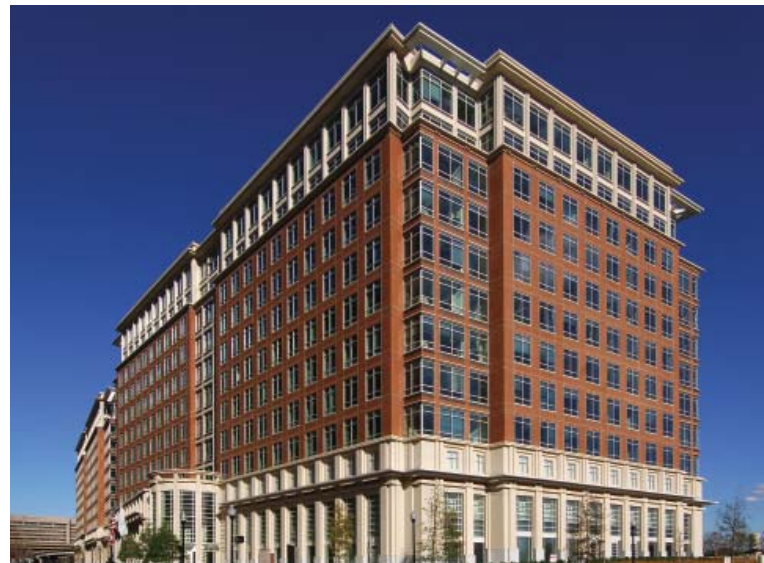
Fig. 3.2—Use of water diversion, architectural details, and overhangs (Potomac Yard – Land Bay A, Alexandria, VA). Photo courtesy of Architectural Precast Association
