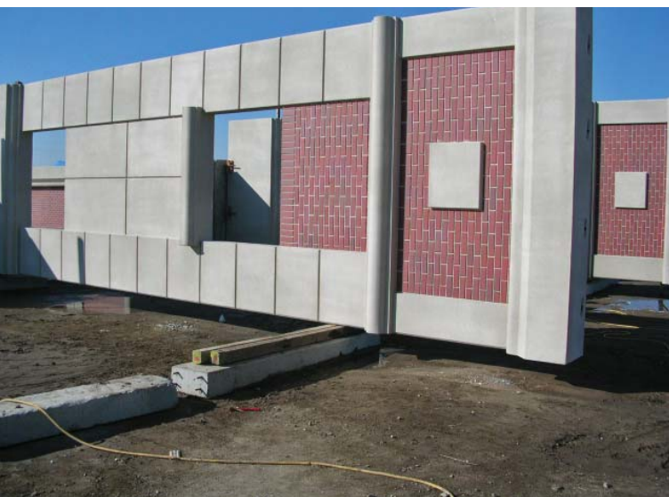
Fig. 3.7—The completed architectural precast panel with all the components included window sills, quoins, and coping. Photo courtesy of National Precast Concrete Association
