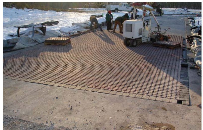
Fig. 3.35—The equipment generally reduces paver installation time by 50 to 70% compared with manual installation. Photo courtesy of Interlocking Concrete Pavement Institute
