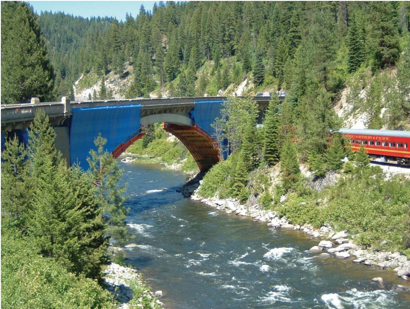
Fig. 4.12—Rainbow Bridge during rehabilitation (Cascade Mountains, ID). Photo courtesy of International Concrete Repair Institute
