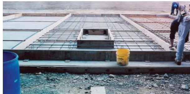
Fig. 1.25—Welded wire reinforcement placement in tilt-up panel. Photo courtesy of ACI Committee 439 volunteers
