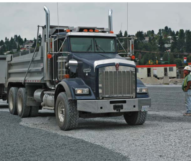
Fig. 3.41—A base layer of No. 56 stone enables a transition between the subbase and bedding layer, causing all stone layers to interlock and “choke” into each other. The No. 56 layer also provides runoff storage capacity. Photo courtesy of Interlocking Concrete Pavement Institute
