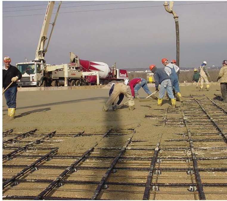
Fig. 3.23—Placing a cast-in-place post-tensioned foundation.
