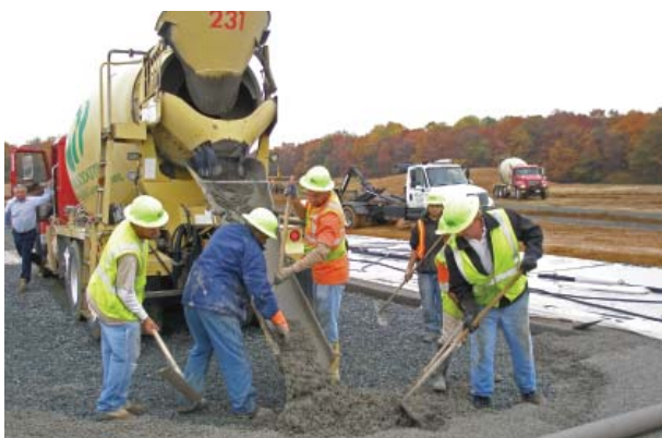
Fig. 3.27—The porous nature of pervious concrete allows water to drain through and recharge aquifers, helping to replenish groundwater supplies. Photo courtesy of Portland Cement Association
