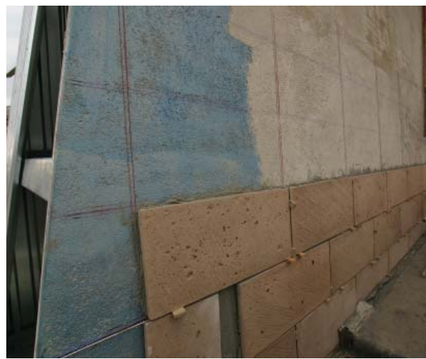
Fig. 3.8—Installation of thin veneer precast on the Mariachi Plaza subway station in East Los Angeles, CA. Photo courtesy of National Precast Concrete Association
