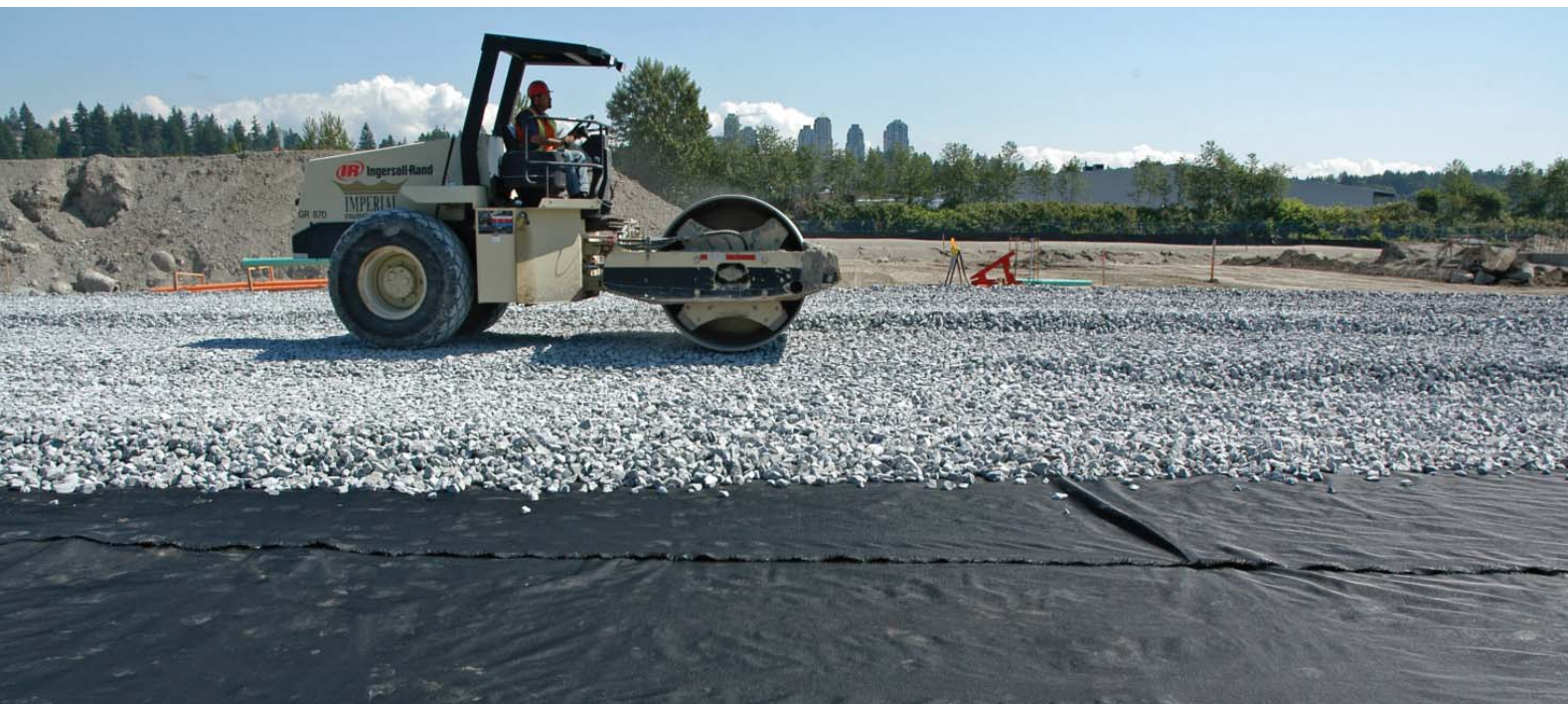
Fig. 3.40—Large stone similar to railroad ballast in size created a stable subbase and ample water storage under the parking lot. Photo courtesy of Interlocking Concrete Pavement Institute
