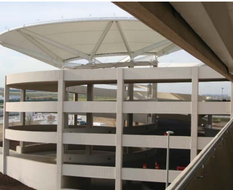
Fig. 1.17—Indianapolis Airport Parking Garage. Photo courtesy of Silica Fume Association
