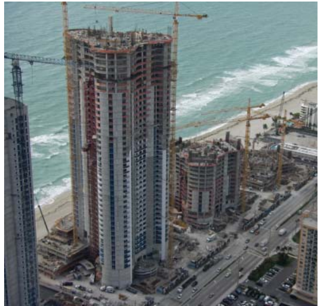
Fig. 2.22—Limited construction site space during construction of the Trump International Beach Resort in Sunny Isles Beach, FL. Photo courtesy of the American Concrete Pumping Association
