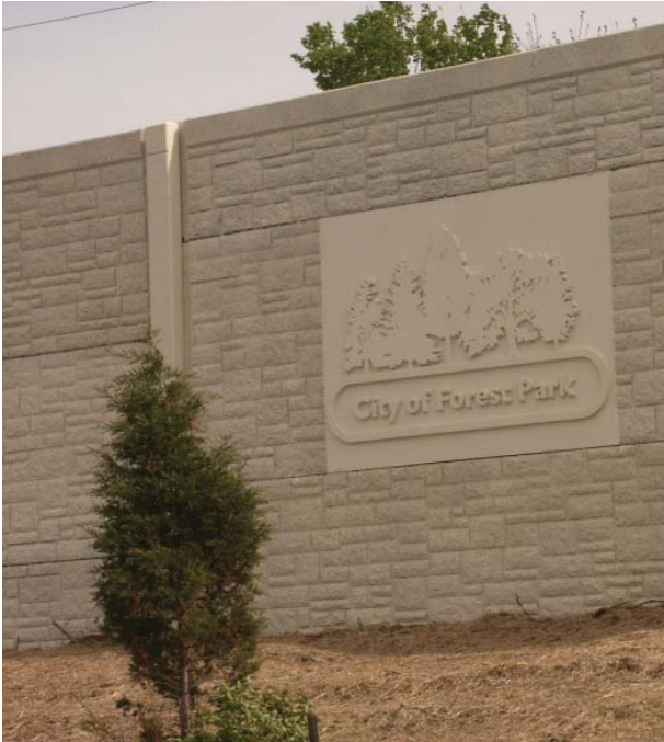
Fig. 3.69—Precast sound wall with decorative features. Photo courtesy of National Precast Concrete Association
