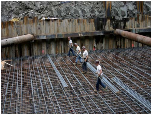
Fig. 1.22—Bar placement in the foundation of the Trump International Hotel & Tower. Photo courtesy of Jack Gibbons, Concrete Reinforcing Steel Institute
