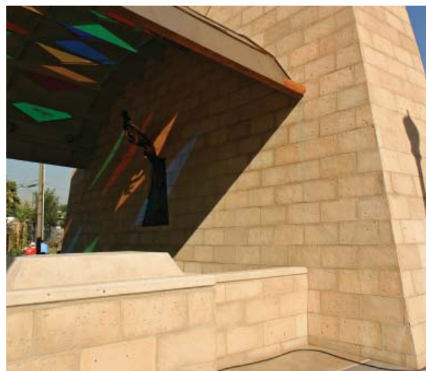
Fig. 3.9—The centerpiece of the plaza is a gazebo created with Mexican cantera stone and donated by the city of Guadalajara in honor of the mariachi bands who congregate in the always-lively plaza. Photo courtesy of National Precast Concrete Association
