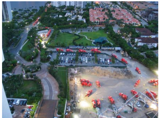
Fig. 2.23—Delivery location for concrete trucks (in red) to pumps (Peninsula II Condos, Aventura, FL). Photo courtesy of the American Concrete Pumping Association
