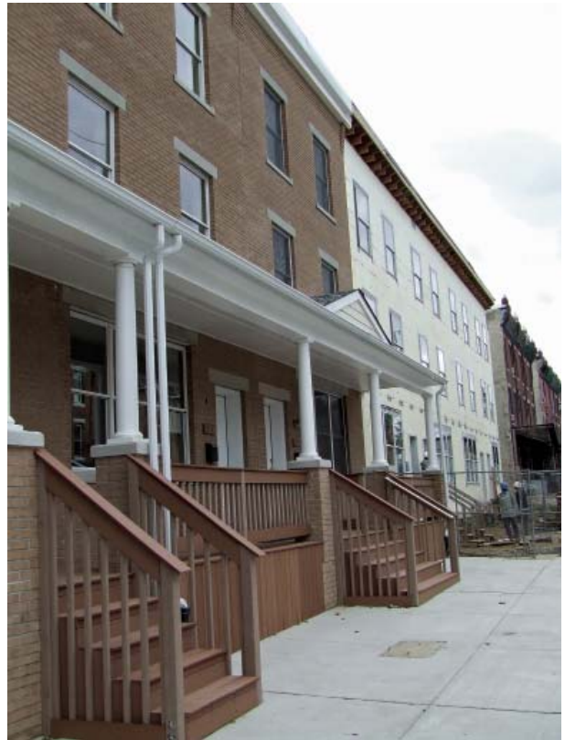
Fig. 3.49—East Parkside residential units. Photo courtesy of Portland Cement Association
