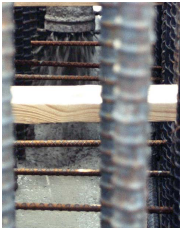
Fig. 1.12—SCC flowing into the reinforcing cage. Courtesy of Silica Fume Association
