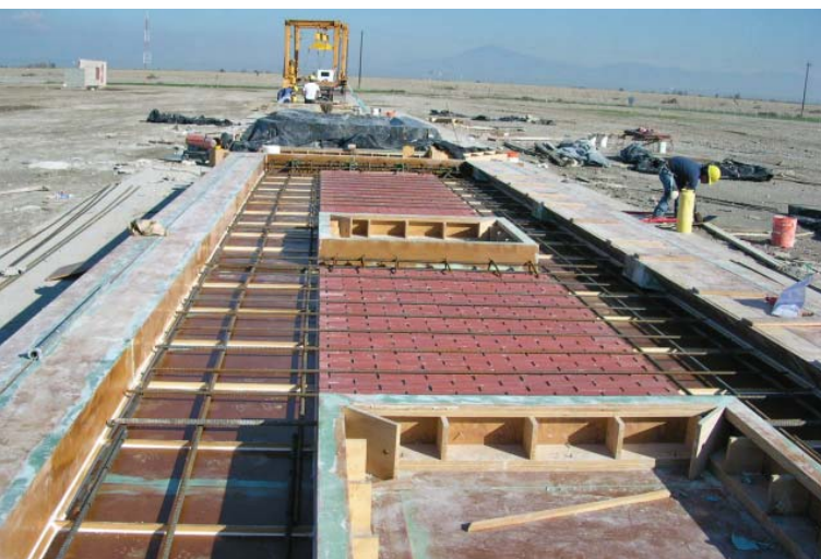
Fig. 3.6—Precast form with thin brick installed in a form. Photo courtesy of National Precast Concrete Association
