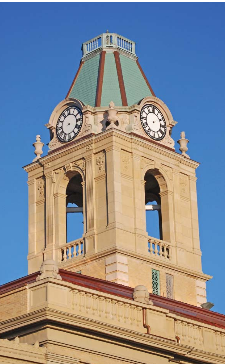
Fig. 3.22—Restoration of decorative detail at Robertson County Courthouse, Springfield, TN. Photo courtesy of Cast Stone Institute
