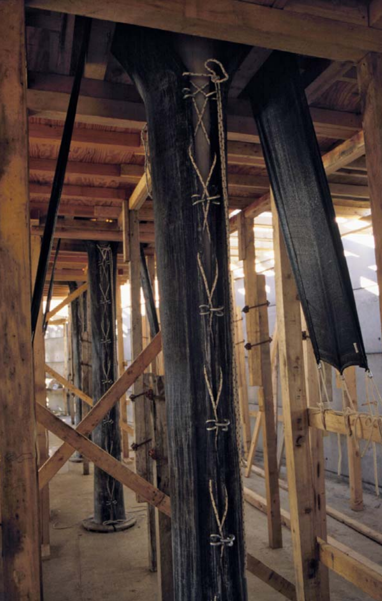
Fig. 2.20—Sample of fabric concrete forms (showing variations in circumference, height, and capital design). Photo courtesy of Mark West
