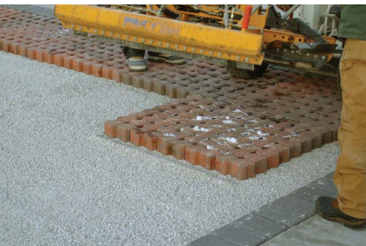
Fig. 3.33—The permeable interlocking concrete pavers are supplied and installed in layers on the screeded bedding material (pea-sized aggregate—bedding sand is never used in PICP). Note the snow on the pavers doesn't interfere with installation, and the border coarse against the concrete curb provides a finished edge. Photo courtesy of Interlocking Concrete Pavement Institute
