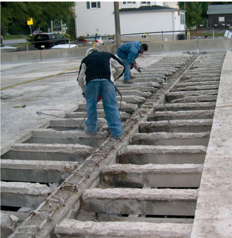
Fig. 4.14—Exposing structural members for repair. Photo courtesy of International Concrete Repair Institute
