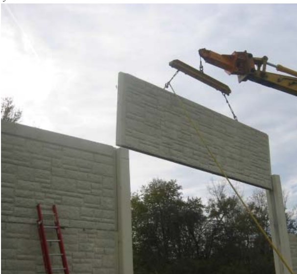
Fig. 3.70—Precast sound wall during placement. Photo courtesy of National Precast Concrete Association
