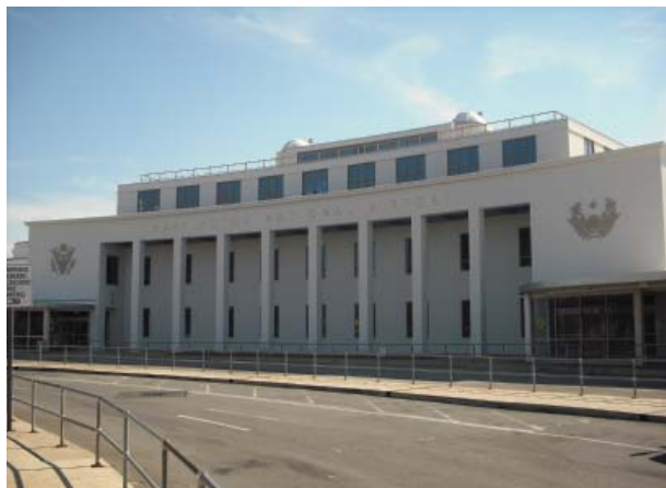
Fig. 4.11—Restored structure. Photo courtesy of International Concrete Repair Institute
