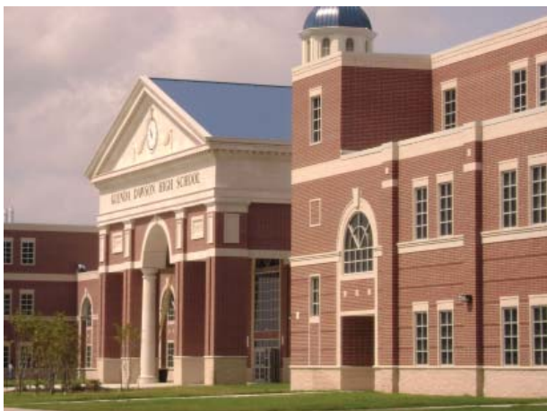
Fig. 3.18—Cast stone allowed the main entrance to become an intricate focal point. Structurally, the columns served as the load-bearing members, and the cast stone was voided out to allow an anchoring system to attach the stone in addition to allowing room for plumbing, electrical, and other mechanical systems. Photo courtesy of Cast Stone Institute
