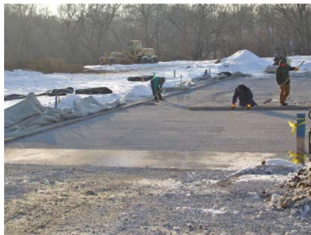
Fig. 3.32—Screeding smooth to receive the permeable pavers. Photo courtesy of Interlocking Concrete Pavement Institute
