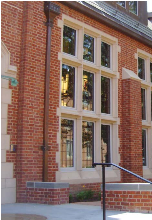
Fig. 3.20—Cast stone used in this collegiate-gothic style building with ornate window and door surrounds at The Taft School in Watertown, CT; and integration of new cast stone into the existing Joule Hotel, Dallas, TX, designed to appear as if it had always been an architectural element (Joule Hotel, Dallas, TX). Photo courtesy of Cast Stone Institute
