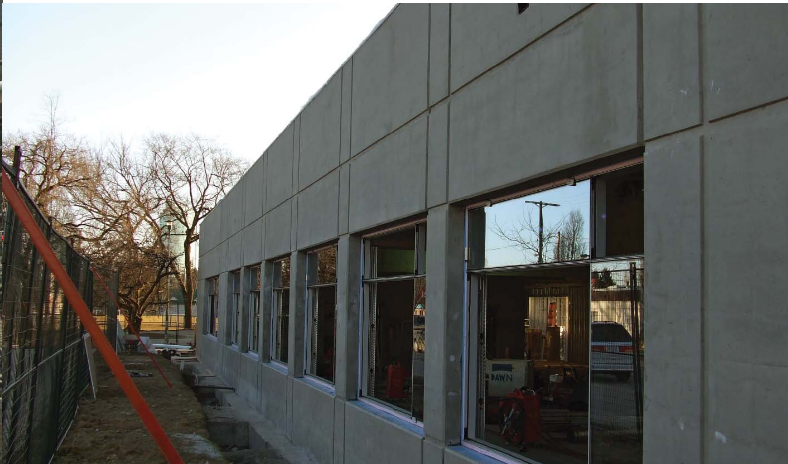
Fig. 3.76—The Surrey Olympic Games Center during construction. Photo courtesy of American Shotcrete Association
