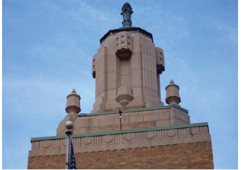
Fig. 3.21—Restoration (before and after): cast stone was used to replicate the entire original exposed aggregate structure, while maintaining the historical integrity of the intricate architectural details (Naples Central School District Naples, NY). Photo courtesy of Cast Stone Institute
