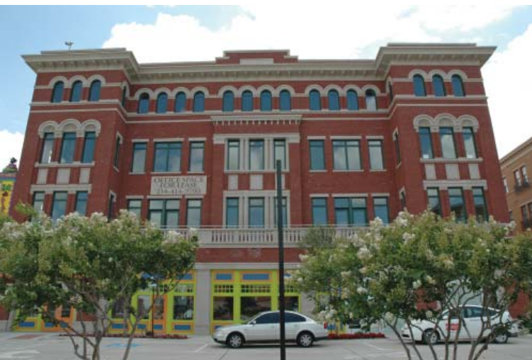
Fig. 3.3—Color and texture to match traditional finishes (Frisco Square Town Center, Frisco, TX). Photo courtesy of Architectural Precast Association
